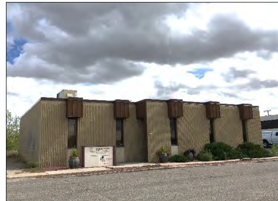
1975, Brutalist office building, 437 S. Spruce St.
