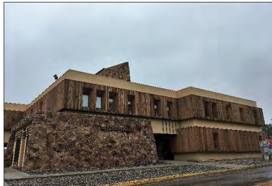
1973 Brutalist building, 167 S. Conwell St.
