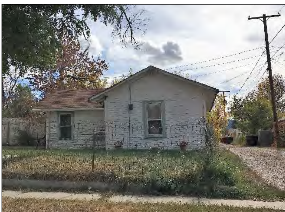
c1920 Intersecting Gable alley dwelling, 711 W. 12 th St.
