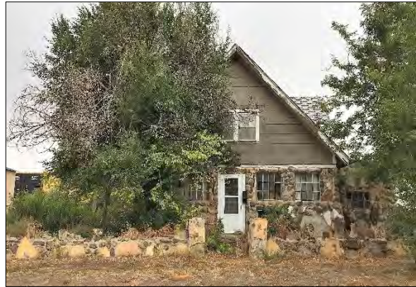
c1918 Gable-Front dwelling, 1220 Burlington Ave.
