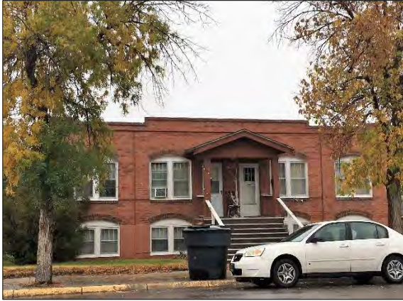
c1924 Four-unit dwelling, 1110 E. 1 st St.
