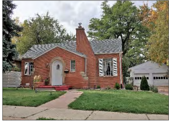
c1936 Tudor Revival dwelling, 1636 S. Spruce St.
