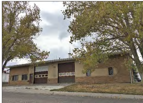
Casper Fire Station No. 6, 280 Valley Dr.
