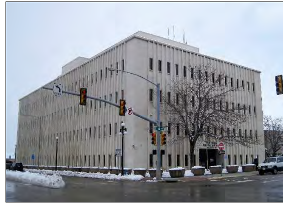
1970 Cheney Federal Building, 100-150 E. B St.
