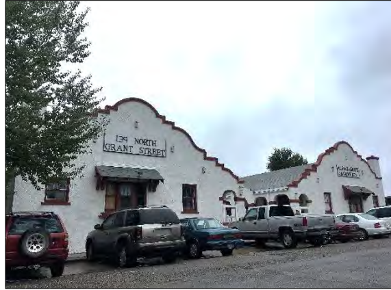
c1920 Multi-Unit building, 139 N. Grant St.
